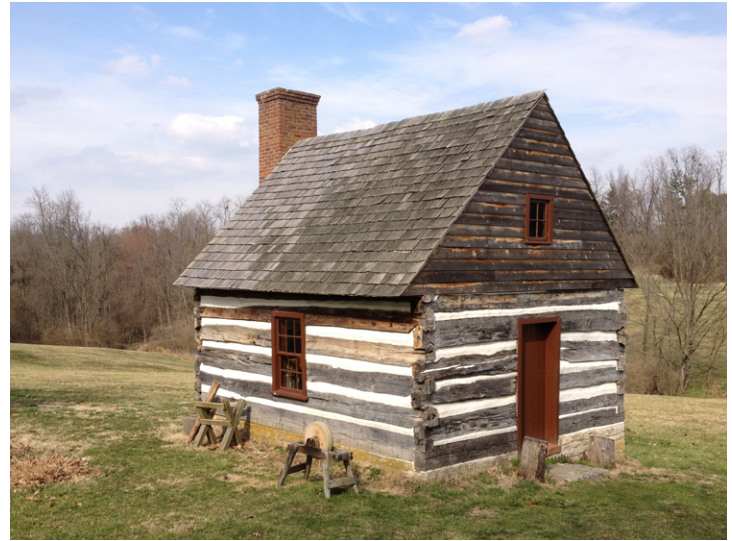
FIGURE 30 - THE WOOD SHOP IS AN EXAMPLE OF AN OUTBUILDING CONSTRUCTED ON EXISTING FOUNDATION WITH OFF SITE MATERIALS
