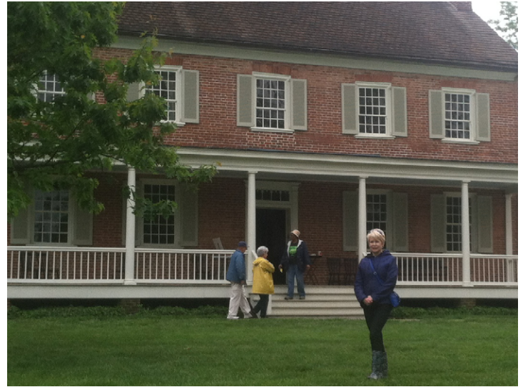
FIGURE 3 - THE NORTH FACE OF THE HISTORIC HOUSE WAS PROBABLY ORIGINALLY THE “BACK DOOR”
