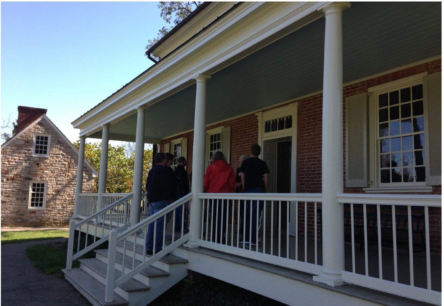
FIGURE 5 - A RAMPED APPROACH ON THE EAST END OF THE PORCH WOULD PROVIDE GREATER ACCESSIBILITY FOR VISITORS
