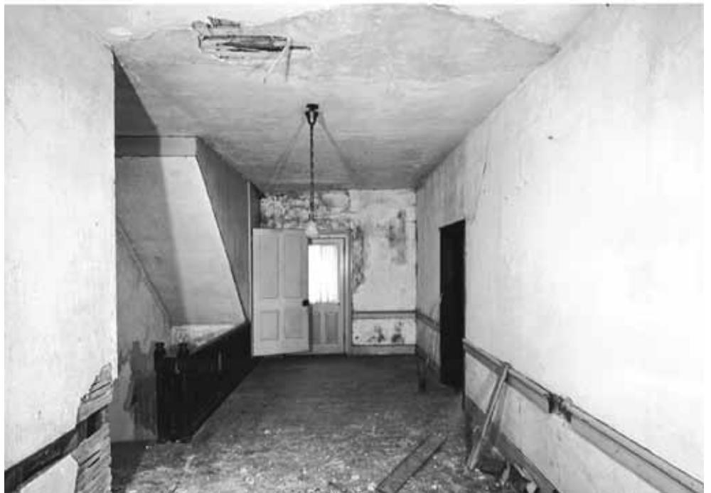
Second floor hall during restoration in 1963
