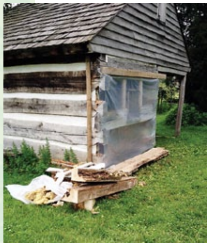
The small shed at the back of the garden is being patched and repaired to prepare for its transformation as the site's new farm distillery.
