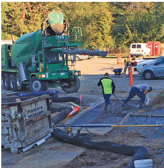
Workers pour concrete for the front entry ramp.
